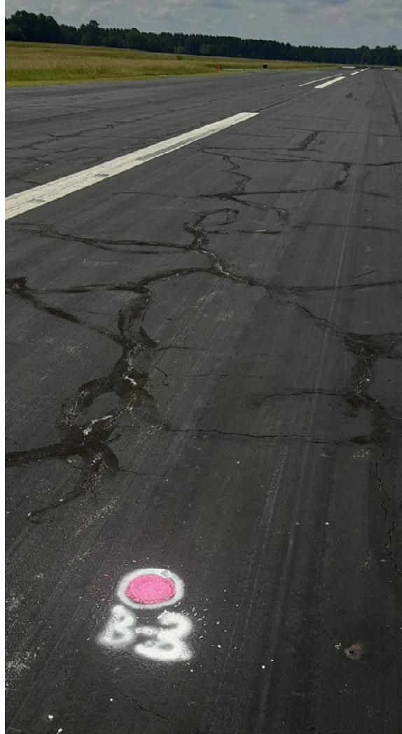
Random cracking, tight block cracking, notable upwelling staining at larger sealed cracks. Bore location 3, looking south.
