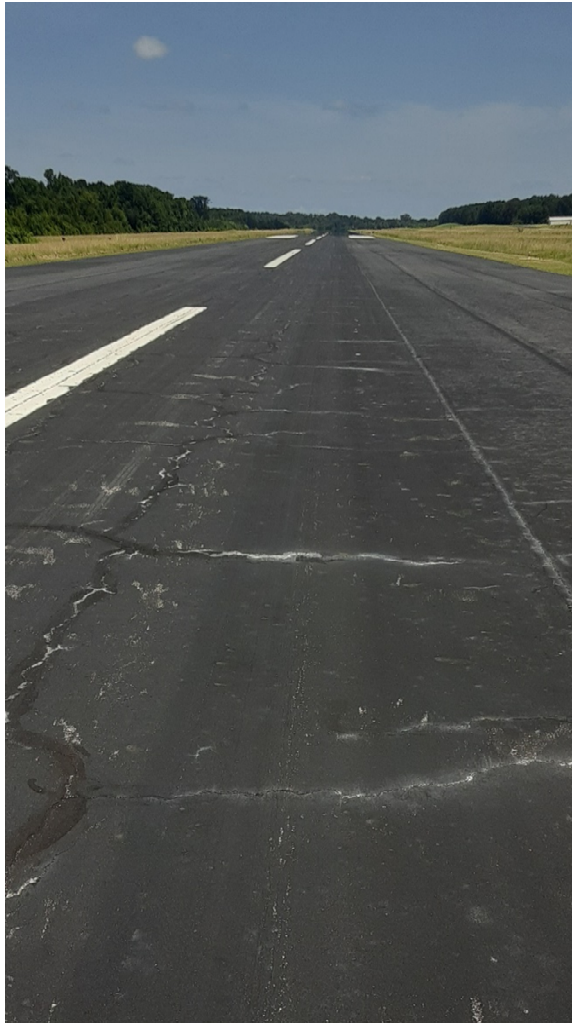
Longitudinal paving joint with staining. Transverse cracks, sealed and unsealed, with staining. Runway 35 approach, looking south.
