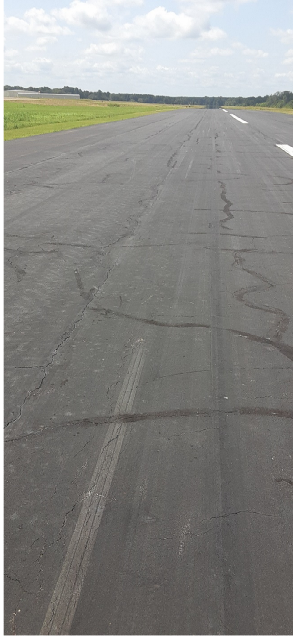
Paving joint cracking, random cracking, crack seal. Notably few stains from upwelling. Runway 17 end looking south.
