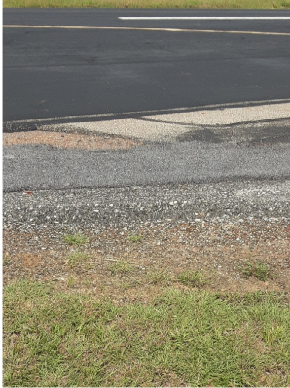
Overlaid pavement layers evident at runway/taxiway connection at south end of runway.
