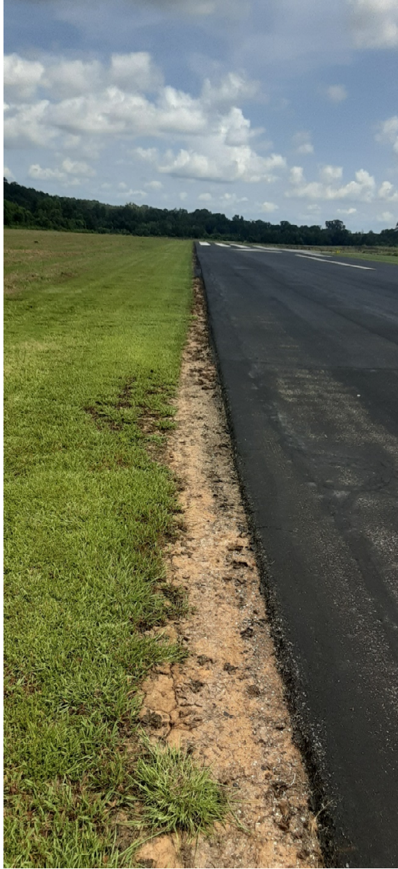
One inch drop off at edge of runway, positive drainage on unpaved shoulder (west side, 17 end, looking north).
