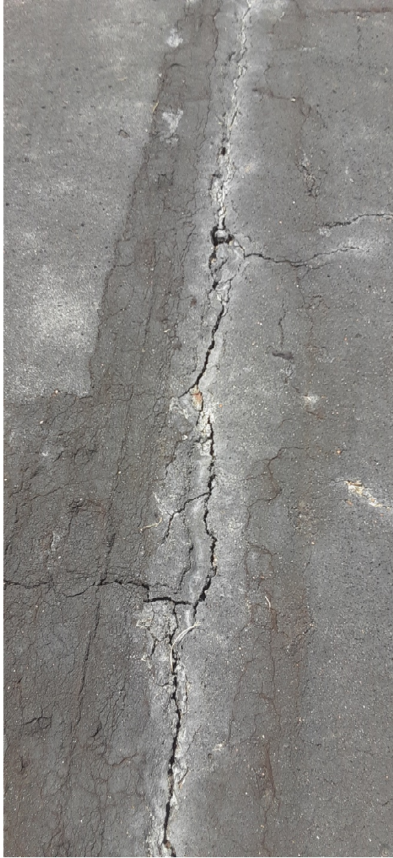
FOD-generating crack adjacent to sealed crack. Evidence of upwelling. South end of Runway.
